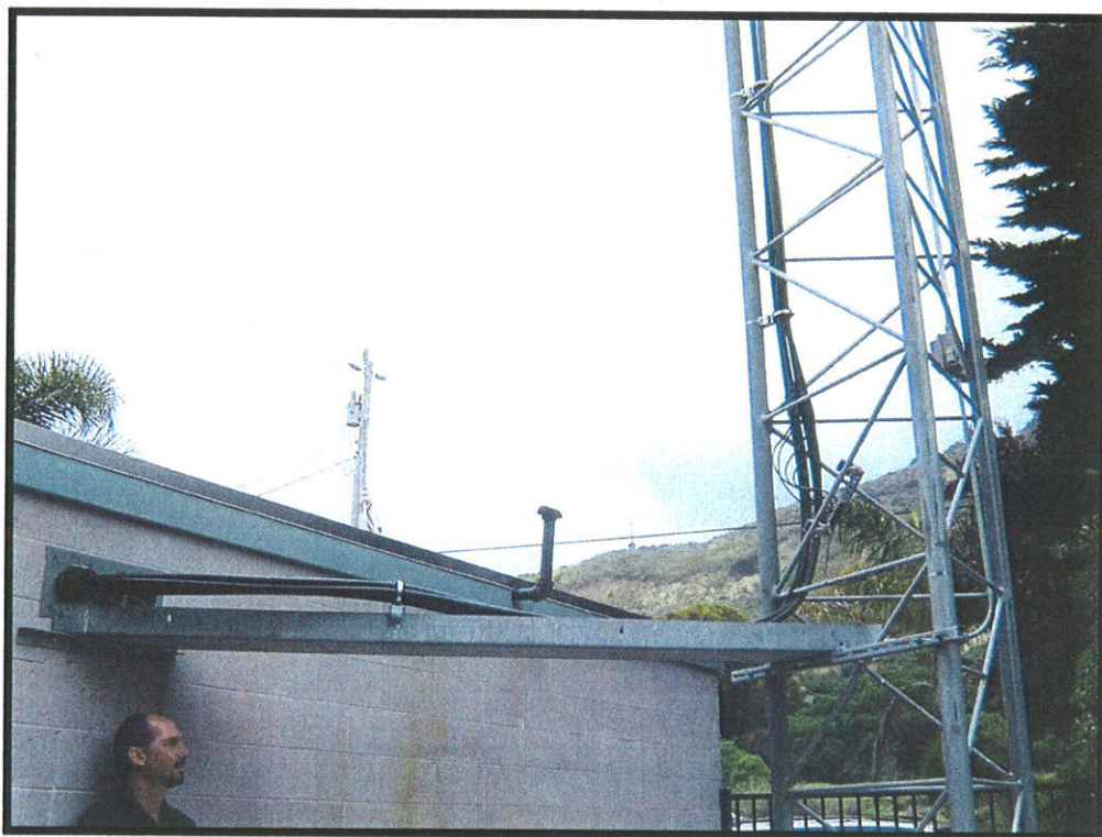
Route waveguide to shelter
