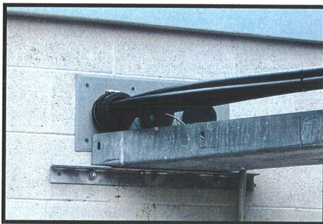
One port was available at time of survey. Likely need to bore more ports.
