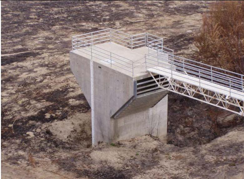
Las Lllajas Detention Basin- Zone 3. Operating Spillway, Reinforced Concrete Two-Way Riser Tower with Projecting Top and Side Inlets with Trash Rack
